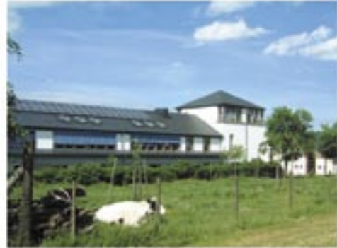
Schoul Heischend 10 kWp/80m 2
